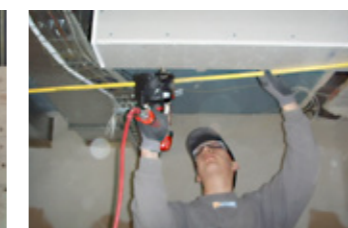
Gypsum board to Metal Stud
