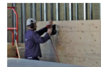
Plywood to Metal Stud
