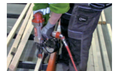
Timber to Metal Stud
