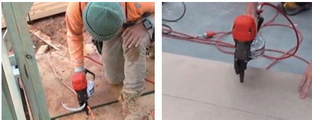
Plywood to Steel
