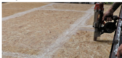
Plywood to Metal Stud
